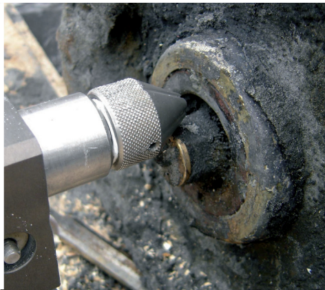
Installation of cutting device
