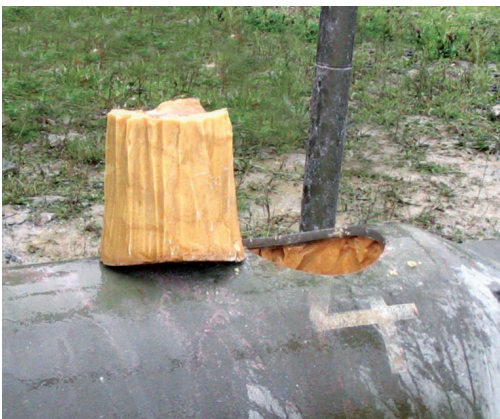
Cutting an access hole (in explosives)
