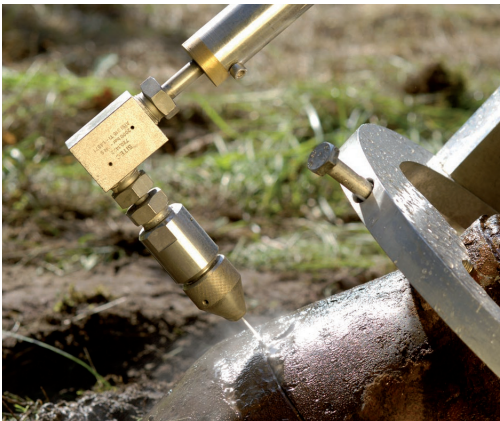
Cutting with Base Fuse Manipulator
