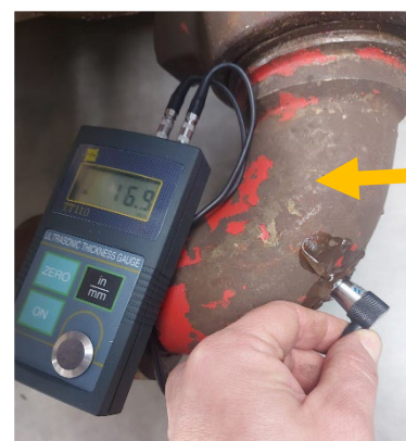
Check for wear by measuring the wallthickness in situ ✓
