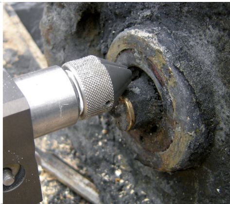
Installation of cutting device
