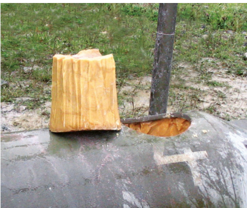
Cutting an access hole (in explosives)
